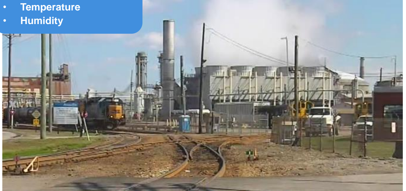
Picture of Cooling Tower Operation used in News Stories
